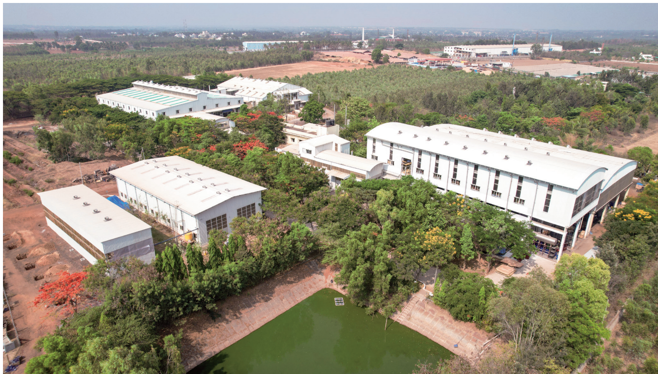
Our Malur manufacturing facility, Kolar
